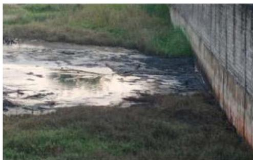
**Figure 4.3: Leakage of liquid waste outside the boundary wall of the CBWTF**
